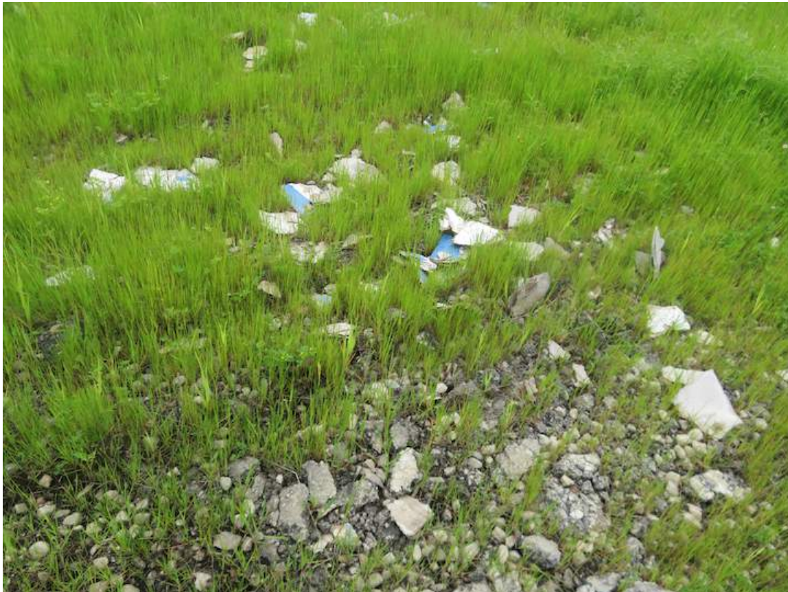
Photograph 13 – Minimal debris, and crushed rock surface.
