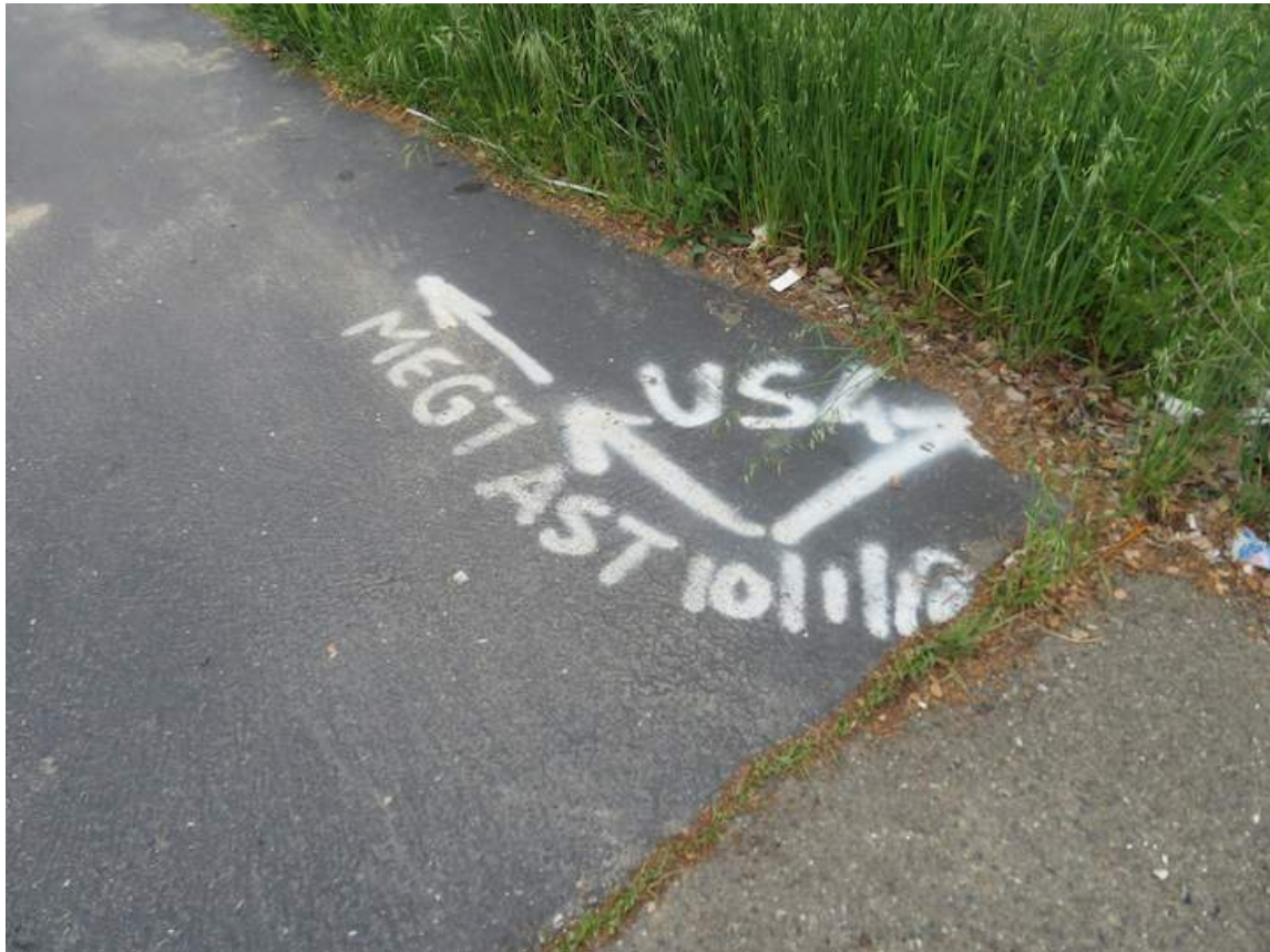
Photograph 5 – Markout for Underground Services Alert.
